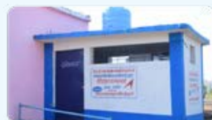
Toilet Reconstruction Work
