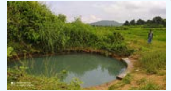
Seepage well constructed at low land
