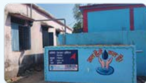
Rainwater Harvesting Unit
