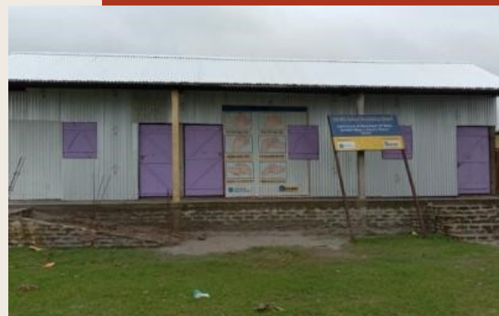
Uttar Schar Lower Primary School, Barpeta district, Assam
