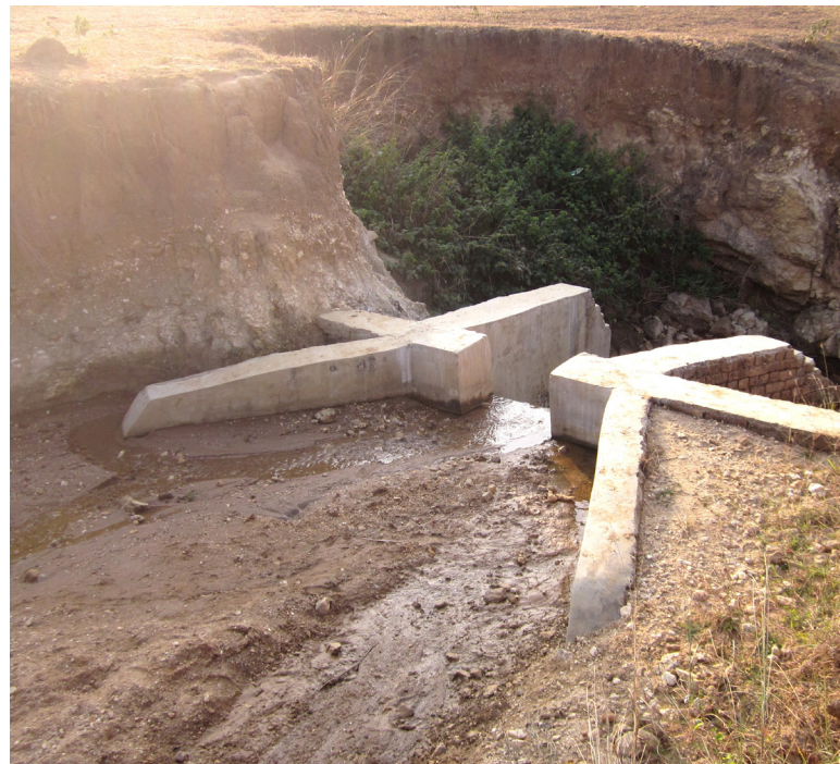
H- Wall check dam (Purnadihi) filled with silt load after first rainy season needs to be cleaned up by the Water User Group for proper functioning next year
