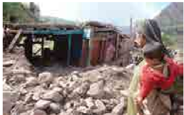
Devastation after the 2005 earthquake at Uri, Kashmir
