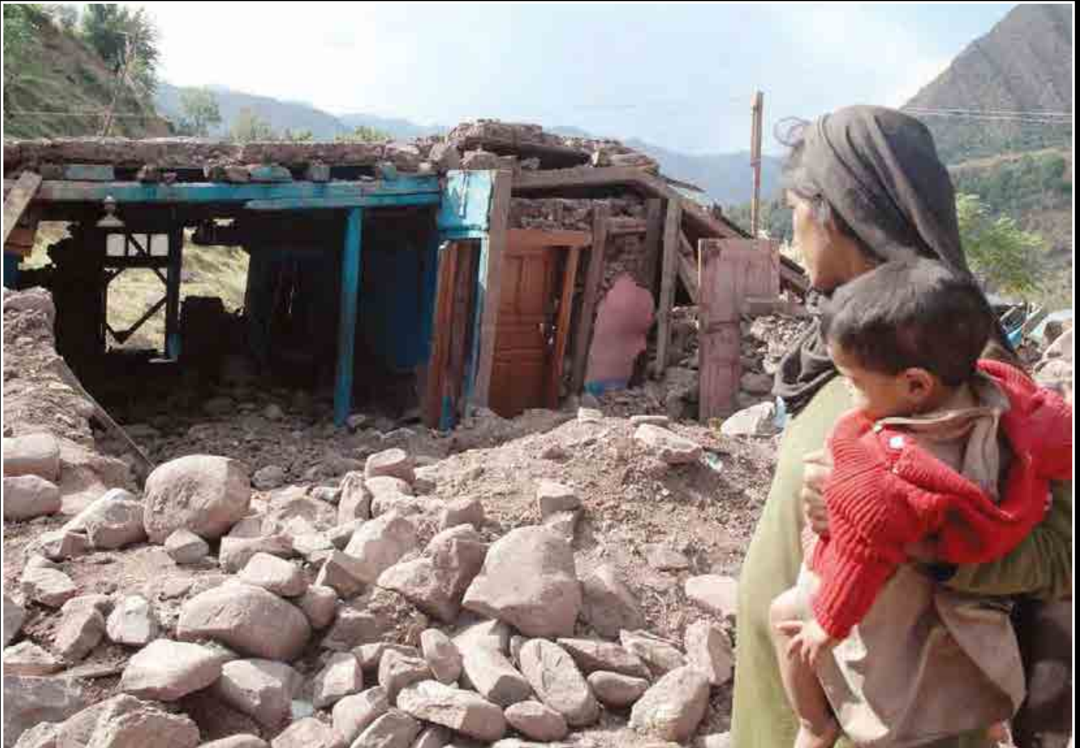
A woman and her child looking at the damage the earthquake caused to their home in Uri, Kashmir. Photo credit: Bilal Bahadur
