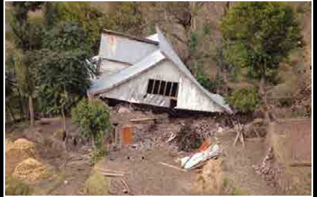
A damaged house after the 2005 earthquake, Uri, Kashmir. Photo credit: Bilal Bahadur
