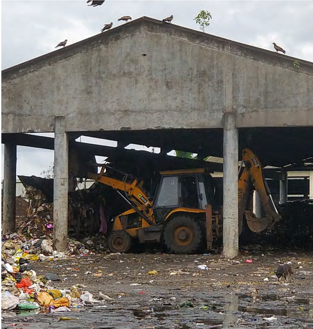
Photo 13 b: MSW Processing Unit- O&M by IL&FS Environmental Infrastructure & Services Ltd, Vidyanayapura
