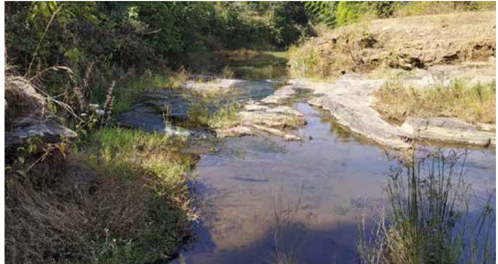
Place identified, and H-Wall Check Dam constructed
