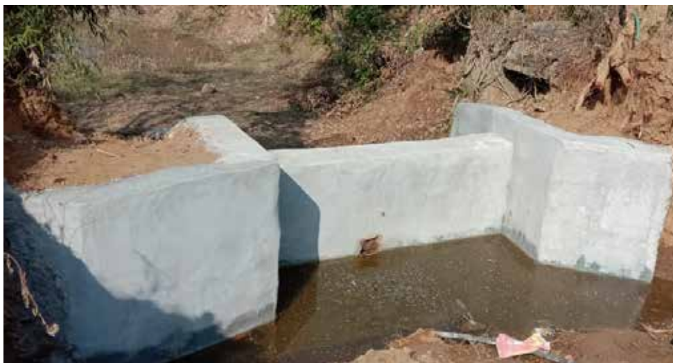
Water level raised to 5 feet after construction
