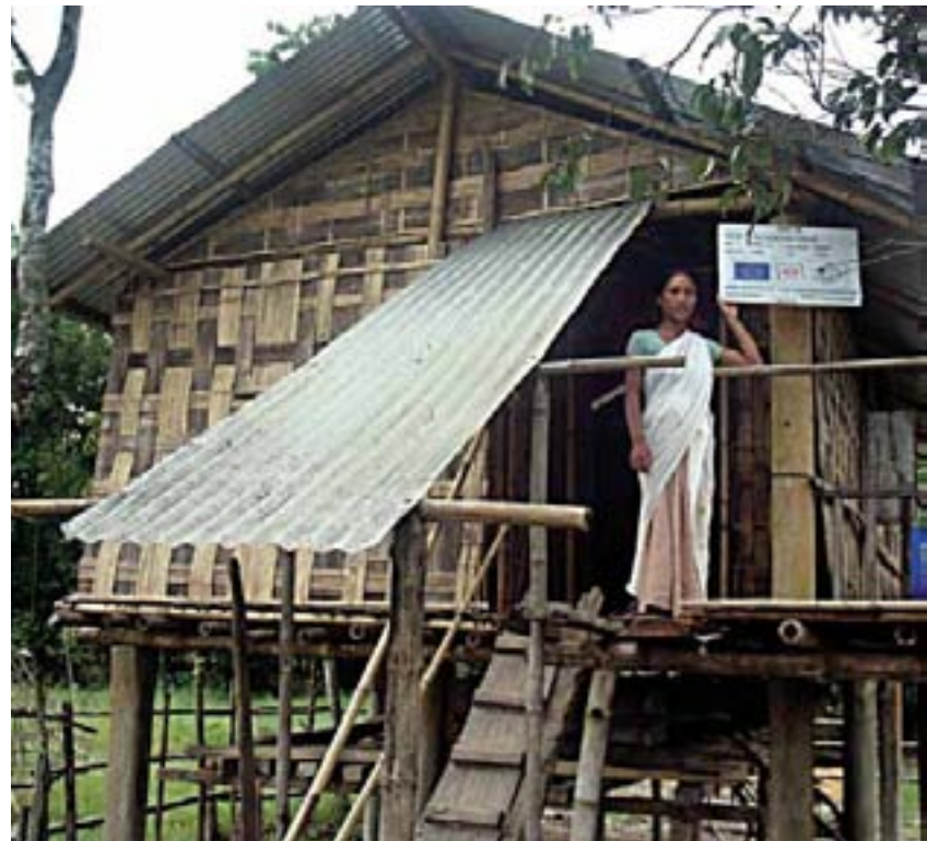
A makeshift high raised house during floods.
