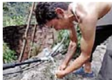
Construction of Public Toilets, Water Tanks and also providing employment under Cash for Work Program was a significant contribution under the program.
