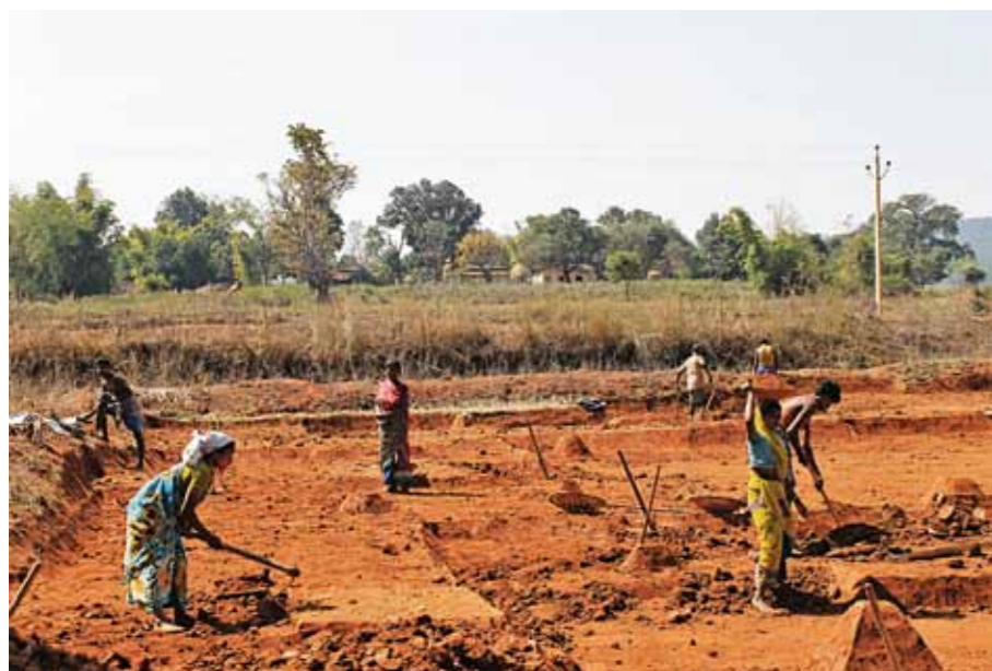
A road construction in progress in North Chhattisgarh.
